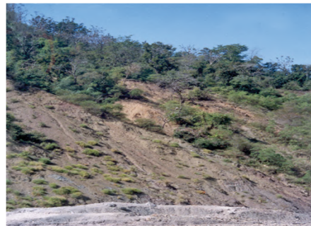
Fig. 2.32: Example of Rotational Landslide
