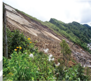
Fig. 2.34: Example of planer rockslide
