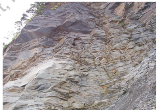
Fig. 2.36: Example of Toppling failure in rocks
